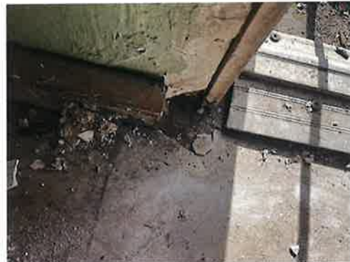
1114-4 12"x12" Floor Tile/Adhesive Interior Laundry Room
